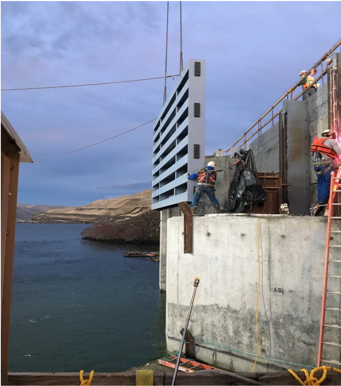
Bulkheads installed. Ready to finish boring hole at bottom of dam.
