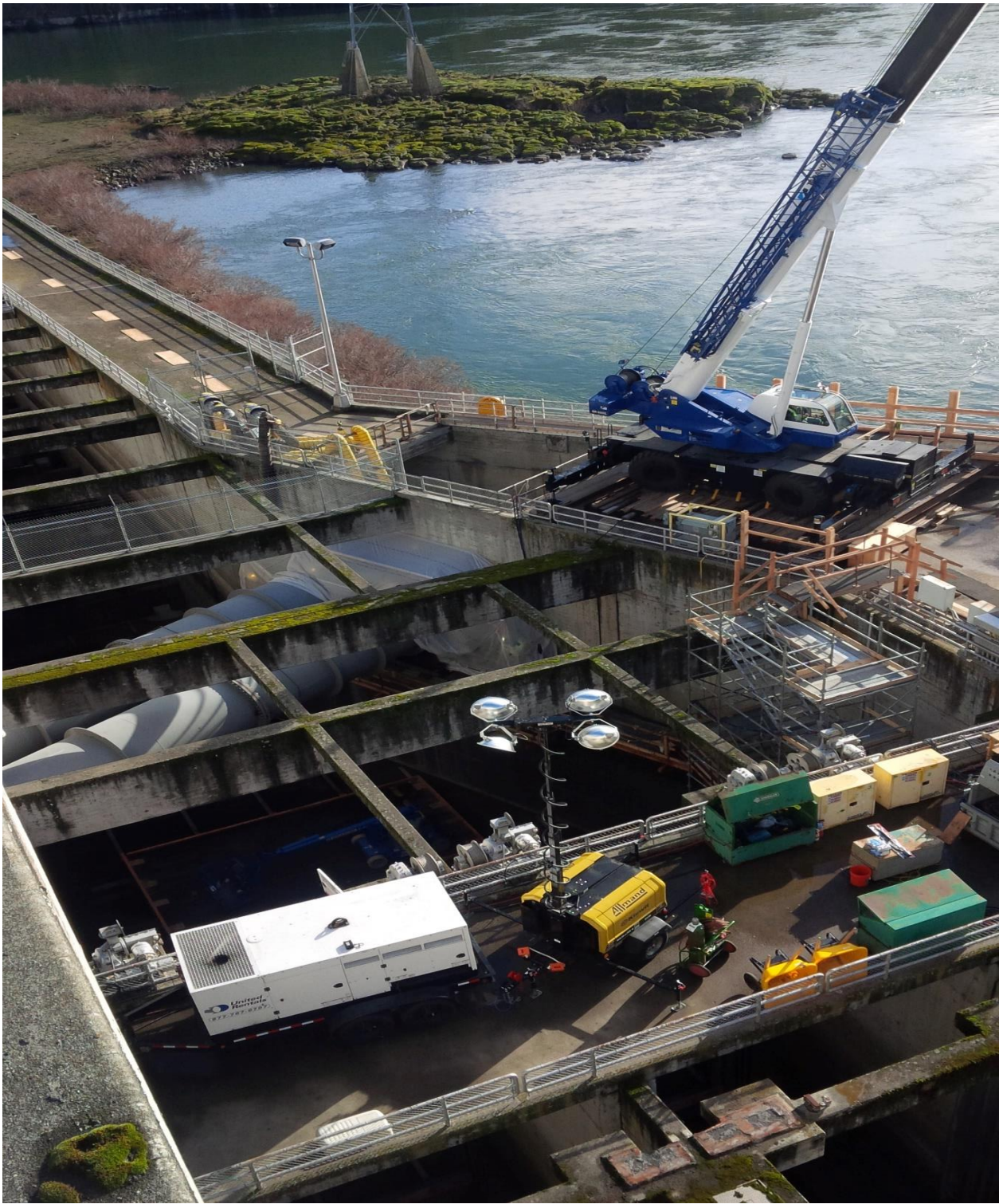
Installing pipe section into AWS chamber.
